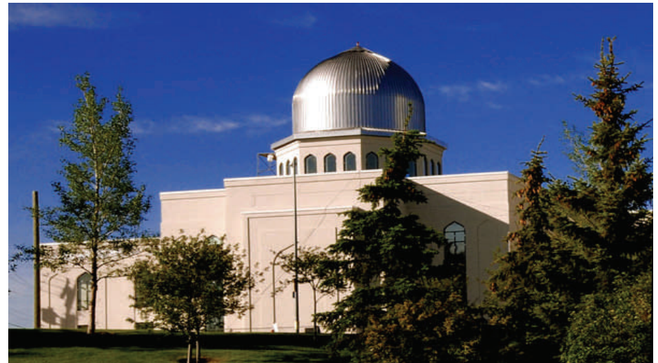
Masjid Baitun Nur Calgary, Canada. The Largest Mosque of Canada.
